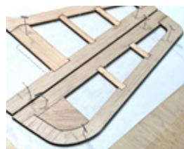
Then glue VF8, VF9 and VF10 in place - again making sure they are all flat and flush.
